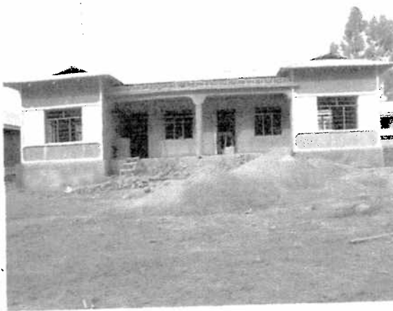
Here is the new administration office building. These offices will house these officers of the school: Director, Principal, Secretary, Treasurer, 2 nd Principal and Academic Master.
