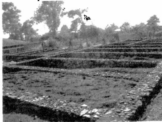
The foundation has been set for the girls' dormitory.
